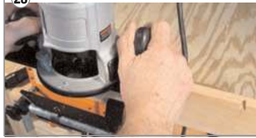
28. Align the layout lines with the centerline in the Top Plate and cut the dovetail sockets.
